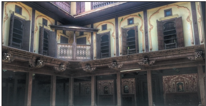
The Phaltan Rajwada is an architectural marvel.
